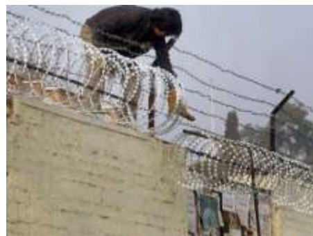
Fig. 19: Concrete walls and barb wires, 2015 Source: The Express Tribune
