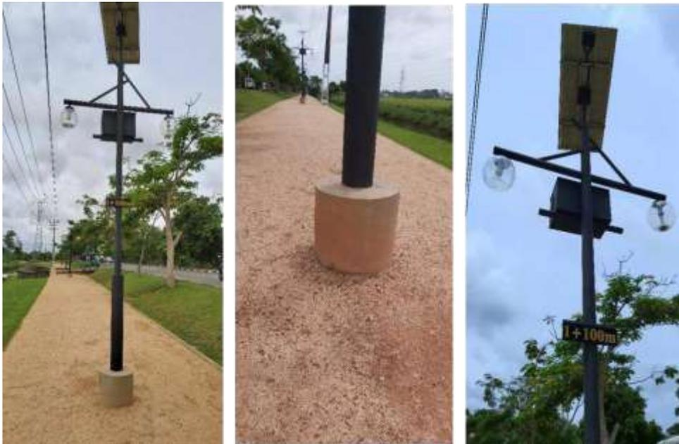
**Fig. 11:** Landscape lighting, position, mounting method and the used materials for the lamp post in Kimbulawela Jogging track
